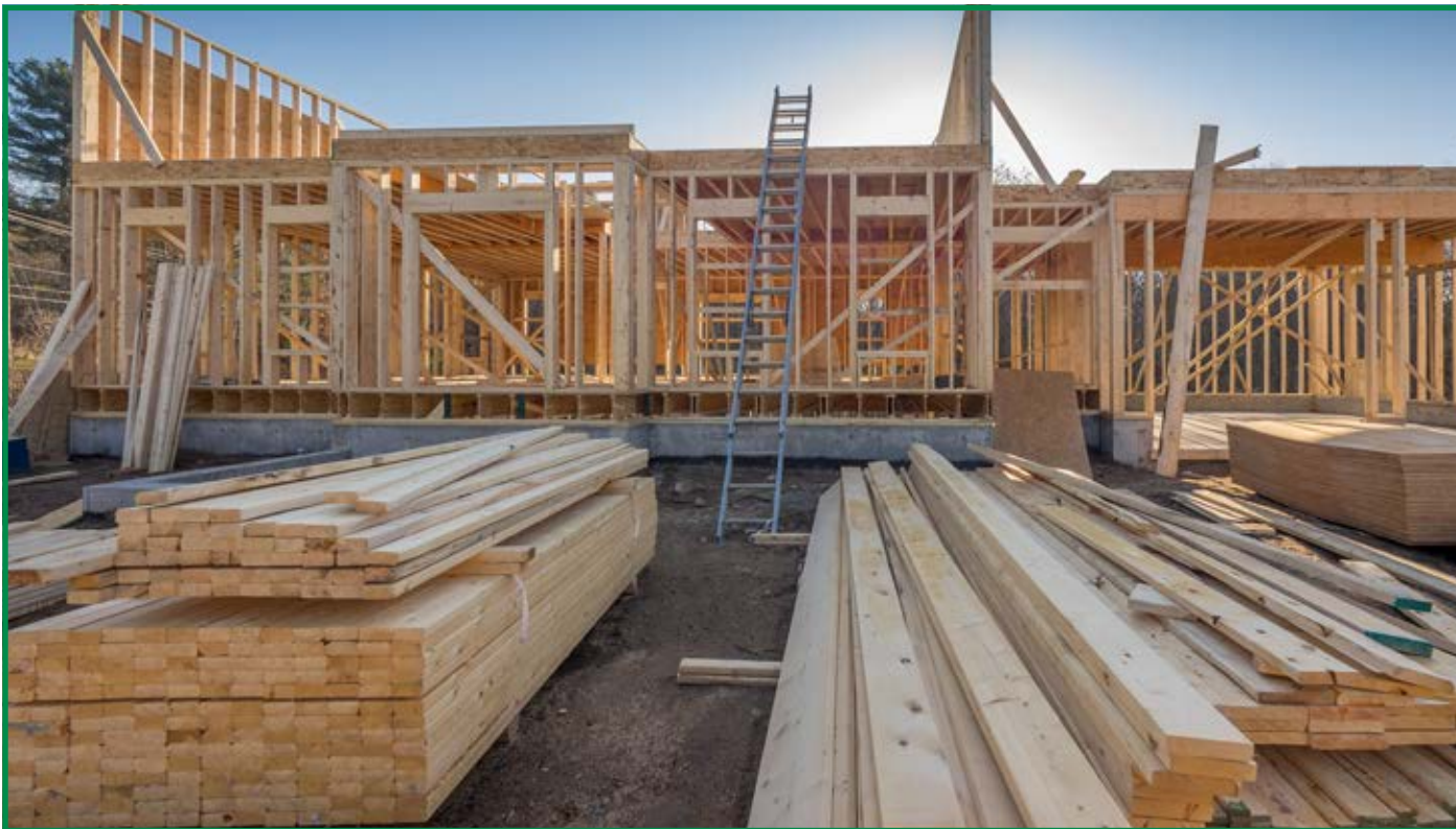
New home construction
